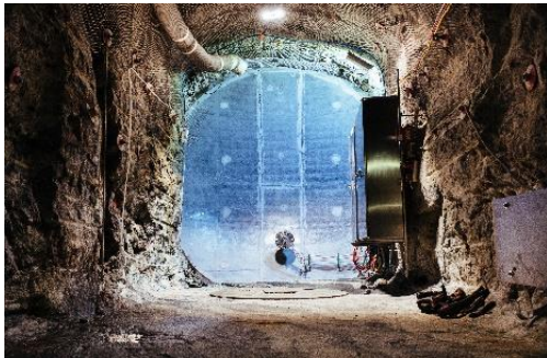
Concrete plug sealing of the demonstration tunnel.
